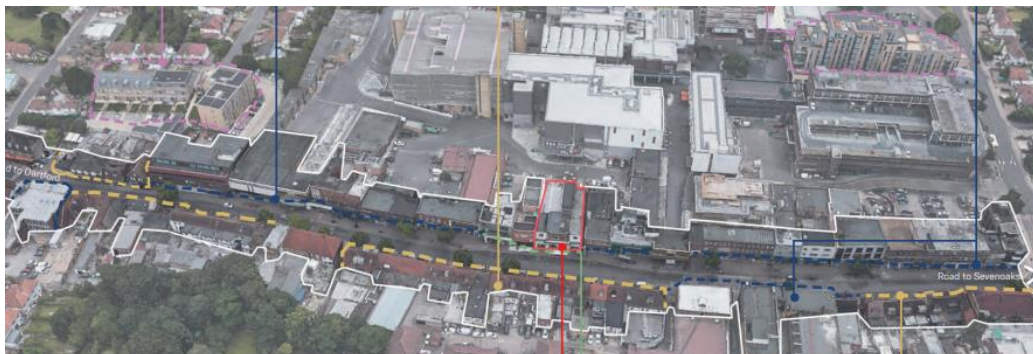
Fig 2. Aerial Photo (site outlined in red)
